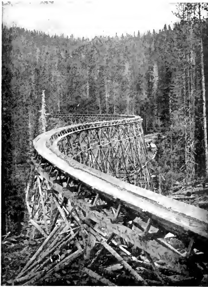
FIG. 159. — A V-flume for transporting Mining Stulls. Montana.
